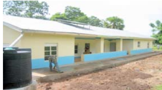
Figure 2: The refurbished building.
