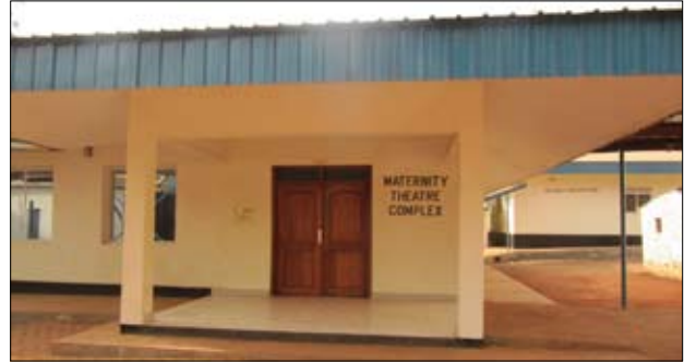
Figure 2. New maternity theatre complex at Wau Teaching Hospital (credit Hilary Fenton-Harris)
