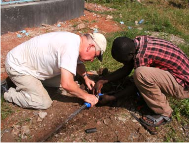
Figure 2. Fixing the plumbing (Nancy MacKeith)
