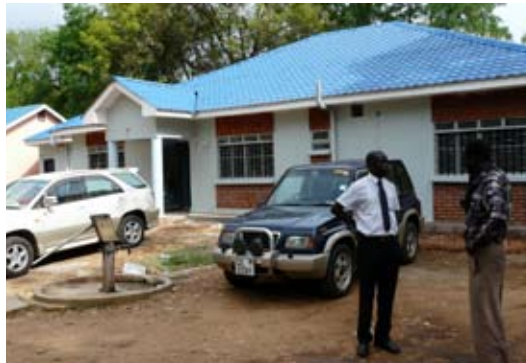
Figure 1 The almost-ready JubaLink Guest House (Credit Eluzai Hakim)
